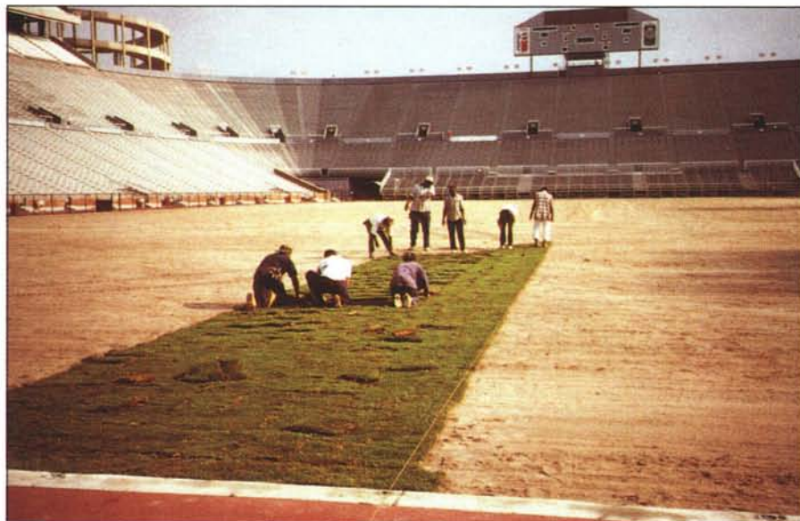
If sod is used, it's very important that any soil on the sod have a very good percolation rate. Photos courtesy: James Boynton III.
