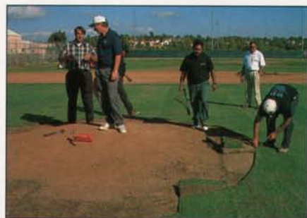
After the sod is laid, the cut-out is made for the pitchers mound.
