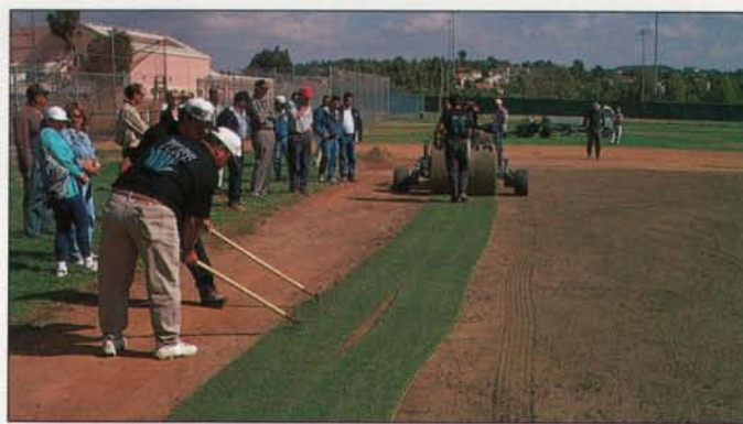
Southern California Chapter members look on as the sodding crew starts laying the infield turf. Photos courtesy: Steve and Suz Trusty.
