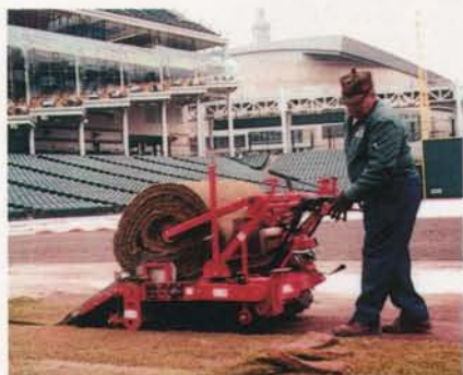
INSTALLED CLEVELAND INDIANS IN 42" AND 48" ROLLS
