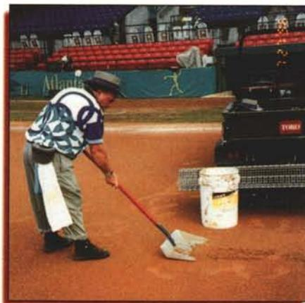
Remove debris, stones and larger size particles while saving infield material and calcined clay. A soil-sifter is a 21st century tool.
