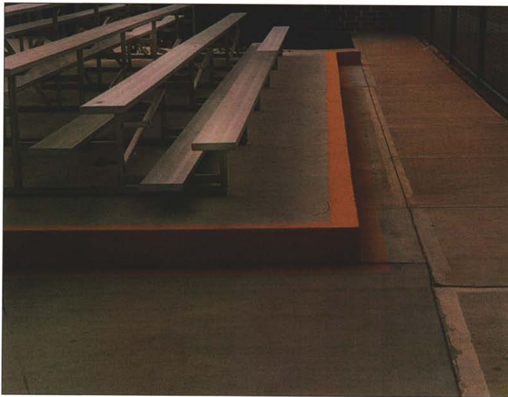
Prudence can be demonstrated at a facility by identifying the difference between two like surfaces; here, yellow paint alerts people to two levels of concrete.
