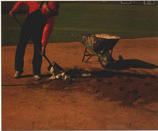
French Drain — Step Three. Fill holes with less dense material, such as sand, pea gravel or small rocks.
