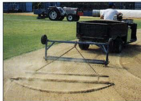
On most skinned ball diamonds, the outer arc will be the area with the greatest problems due to the movement of material during repeated preparation of the area with scarifiers and drags.
