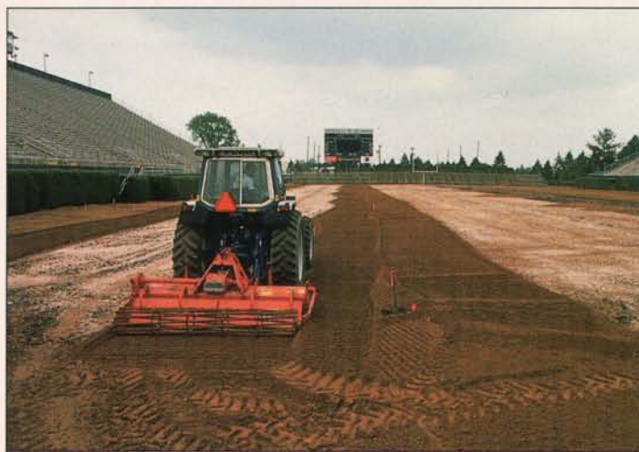
An inorganic soil amendment — a calcined “diatomaceous earth” — was incorporated into the field to help reduce compaction, encourage deep rooting and improve water retention during dry spells.
