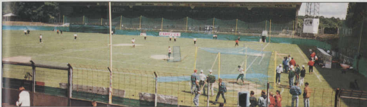
Conversion of Offenbach Stadium called for construction of dugouts, all netting and fencing, a warning track, batting practice equipment, mounds and goal posts for football.
