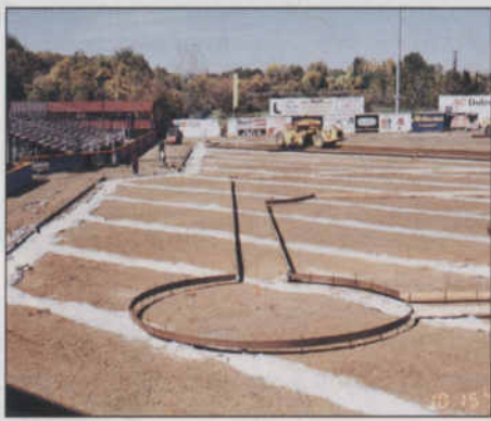
The infield takes shape atop a new drainage system.
