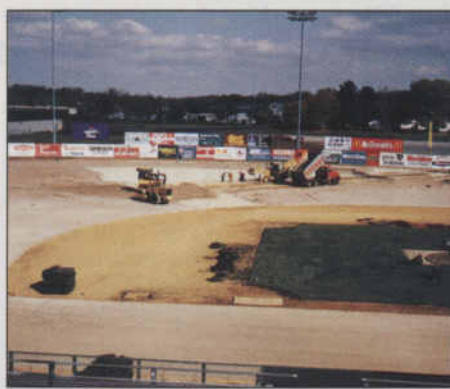
While the infield was being sodded, the nine-inch-deep rootzone for the outfield was prepared.
