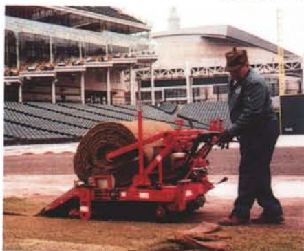
INSTALLED CLEVELAND INDIANS IN 42" AND 48" ROLLS
