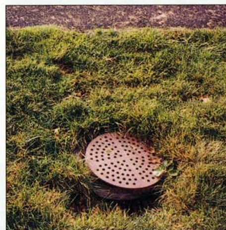
It's important to inspect all catch basins around the field. This kind of situation endangers players.
