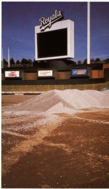
Pea gravel was spread four inches thick over the entire playing field except for the basepaths, home plate and the pitcher's mound. Photo courtesy: Vermeer Manufacturing Co.
