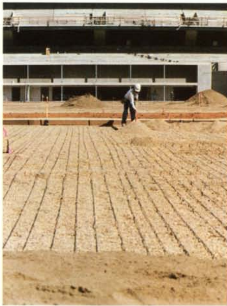
Coors Field in Denver, home of the Colorado Rockies, has 45 miles of underground heating cables installed in the rootzone. Photo courtesy: Randall & Blake, Inc.
