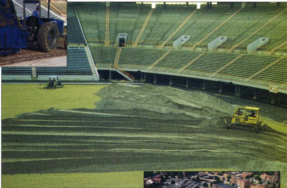
Nutri-Turf sprigged Neyland Field with Tifway 419 (top). The rootzone consists of 90% sand and 10% reed sedge peat. Neyland Stadium in days of artificial turf (right).
