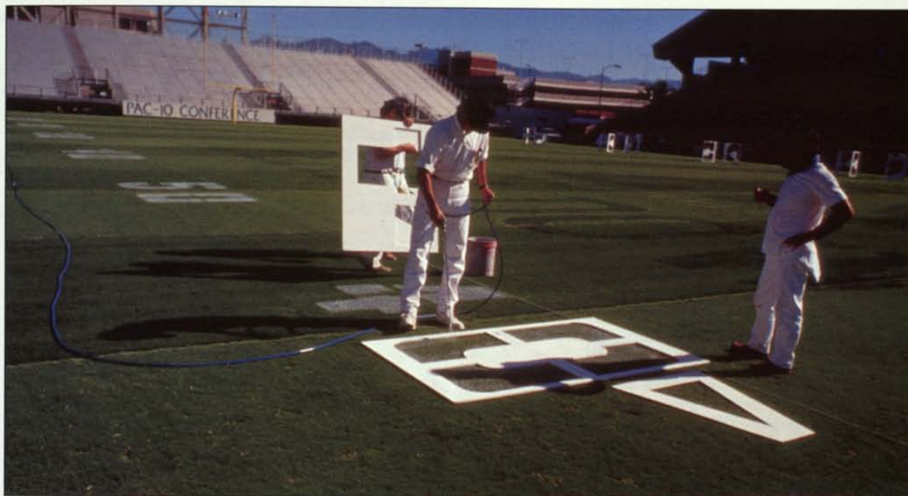
As numbers are painted individually using airless sprayers and custom made stencils.
