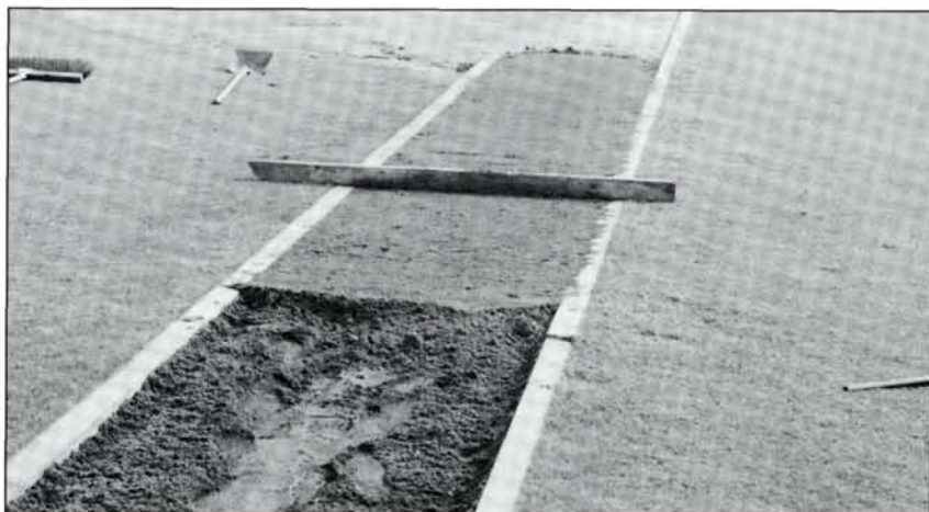
New clay added and leveled after the existing clay has been roto-tilled.
