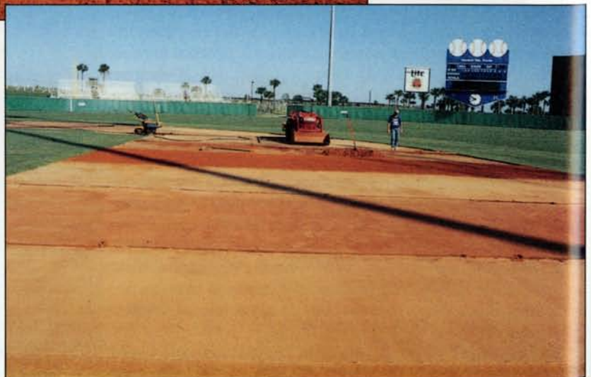
(below) Finish one section at a time until the entire skinned area has been renovated.
