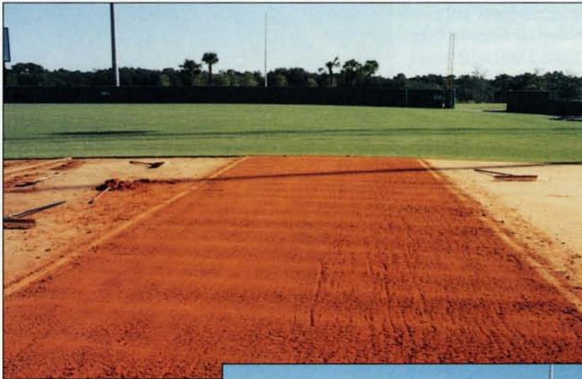
(left) Once the clay has been leveled, as shown here, the next step is rolling.
