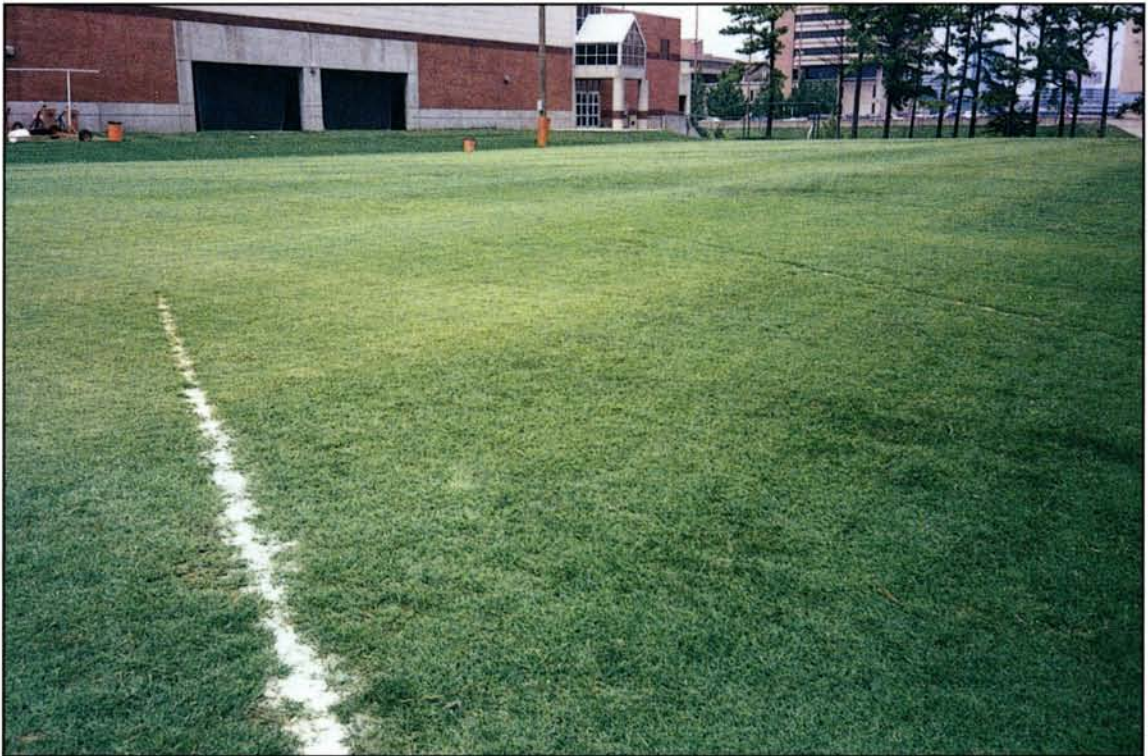
Trench drains installed on a football practice field at the University of Tennessee.
