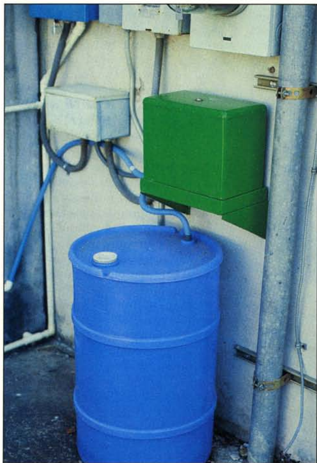
The ability to supplement irrigation with iron, wetting agents or micronutrients through an injector system, can tremendously boost the control a manager has over growth and maintenance of turf. Photo courtesy: Amiad U.S.A., Inc.
