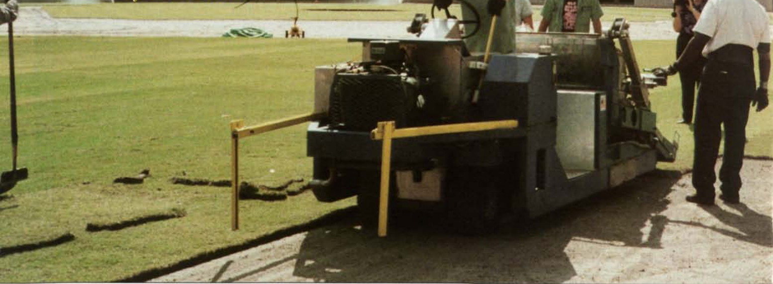
A Cynet 48 turf-installation machine was used to install the baseball field for the Florida Marlins at Joe Robbie Stadium. Photo courtesy: Cynet Turf.
