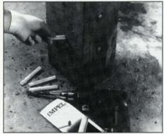
IMPEL Rods are molded from waterdiffusible boron, a natural element recognized as an effective deterrent to rot. The resemble glass rods and are inserted into small holes drilled in wood where it is most susceptible to rot.
