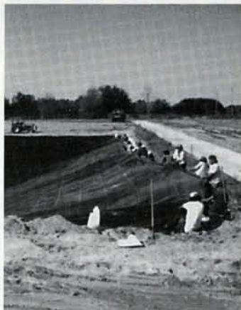
STORMWATER RETENTION POND
