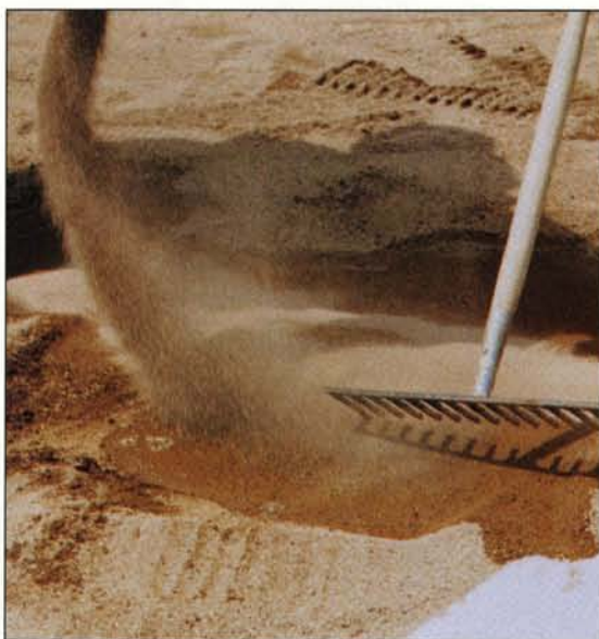
Absorbent calcined clay products, such as Quick Dry, shown in application here, can be used to dry up shallow puddles. Photo courtesy: Aimcor.
