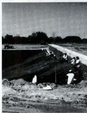
STORMWATER RETENTION POND
