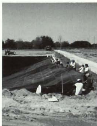
STORMWATER RETENTION POND
