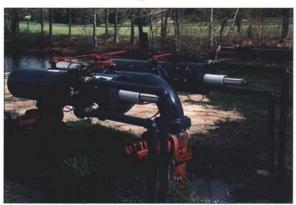
Orival-Filtomat® filters protect sprinklers, mini-jets, drippers, etc. by removing sand, gravel, algae, pollen, silt, leaves, snails, mussels, and other dirt particles down to 15 micron from all types of water. Self-cleaning without interrupting system flow. Require only routine maintenance, no changing of media. Single units handle flow rates to 4800 GPM. Easy to install. Payback usually less than one year. For a free video cassette, contact:
