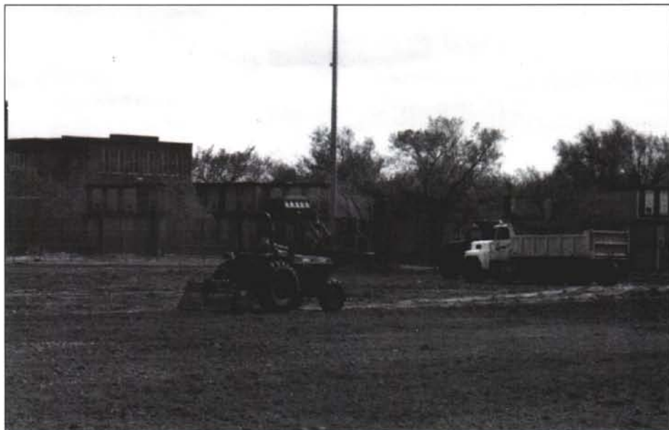
Topsoil installed by one contractor was removed and a new seed bed was prepared.
