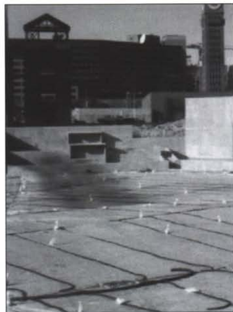
PAT lines over the polyethylene liner. Photo courtesy Don Roberts, STN Sports/Southern Turf Nurseries.
