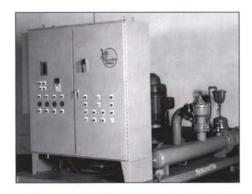
SyncroFlo's Eagle VFD (variable frequency drive) series of pumping stations are designed specifically for the irrigation system. Pump station operation is automatically optimized for peak load requirements with a built-in PC logic controller, which saves energy and operator training.
