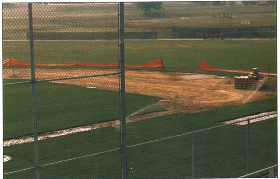
Redbird Field infield under construction.
