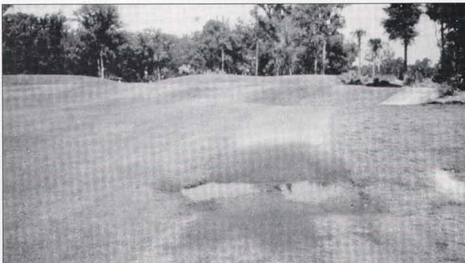
Cart paths present serious drainage challenges and often require renovation.
