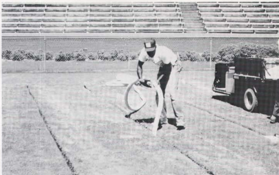
Perforated drainpipe being installed at Jordan Hare Stadium.
