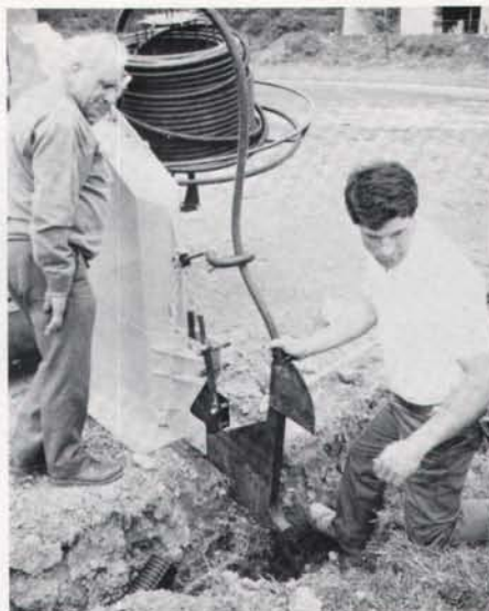
Geoffrey Davison (left) and Joe Motz (right) connect cross-field drain tubes to side line drainpipe.
