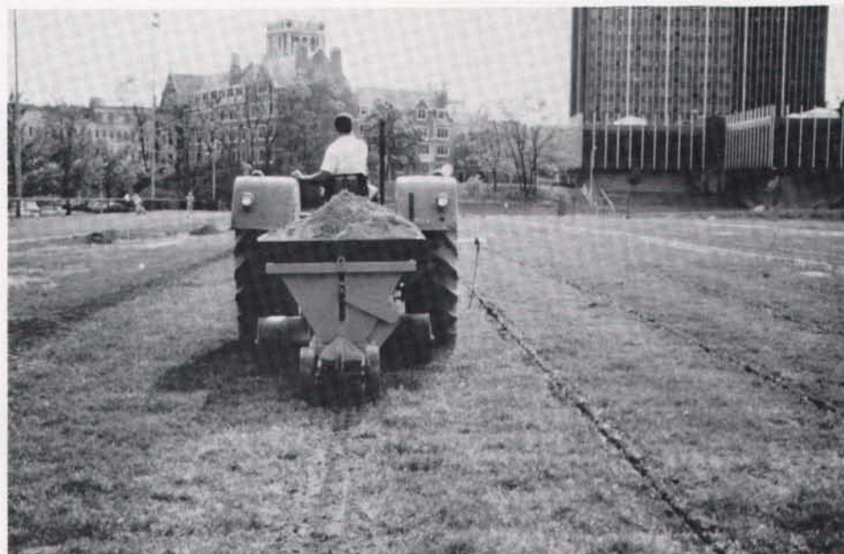
Second device backfills narrow trenches with sand.
