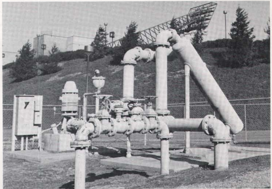
Downstream sand separator at a sports complex removes sand and grit. Photo courtesy: Lakos.
