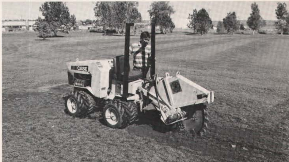
Wheel trencher adapted by Clark cuts narrow trenches up to 18 inches deep.
