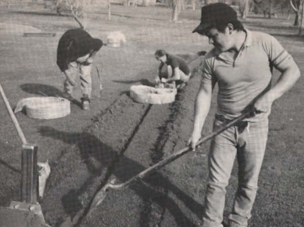
Clark's crew installed more than 8,000 feet of vertical drainpipe in less than two months.
