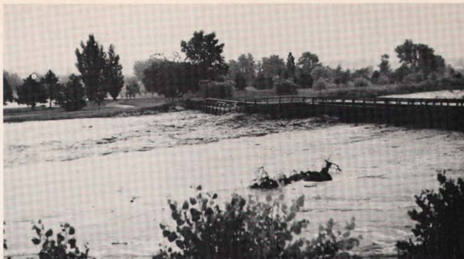
Earthen dike holds back Cherry Creek during flood.
