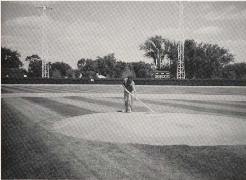
The mound is constructed of blue clay. Mats are buried underneath the mound and home plate to prevent players from creating deep holes.
