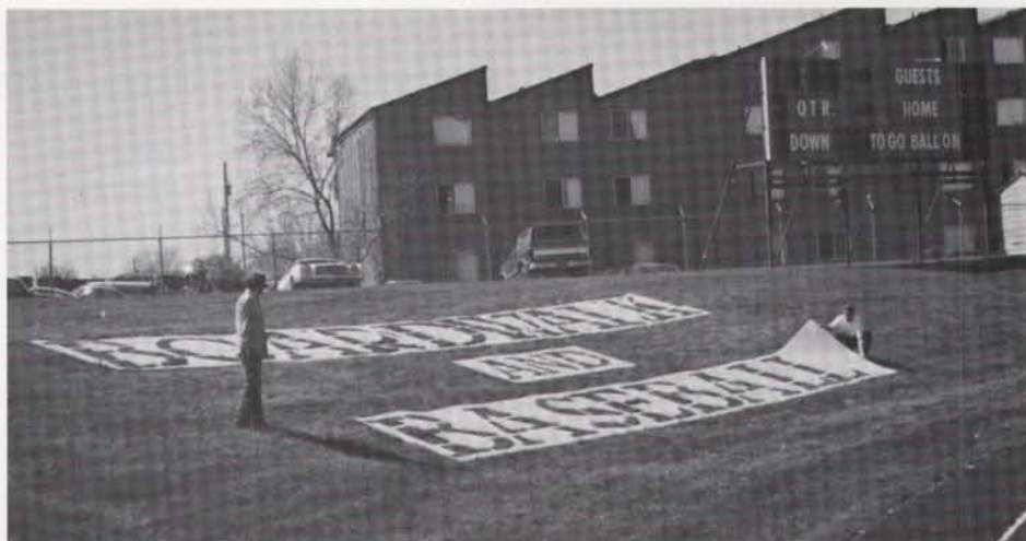
Stencils in place for painting bank at Baseball City, FL, spring training center for the Kansas City Royals. Photo courtesy: Newstripe, Inc.
