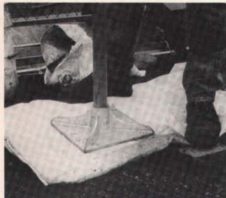
Place a plastic bag over the wet clay to prevent it from sticking to the tamper.
