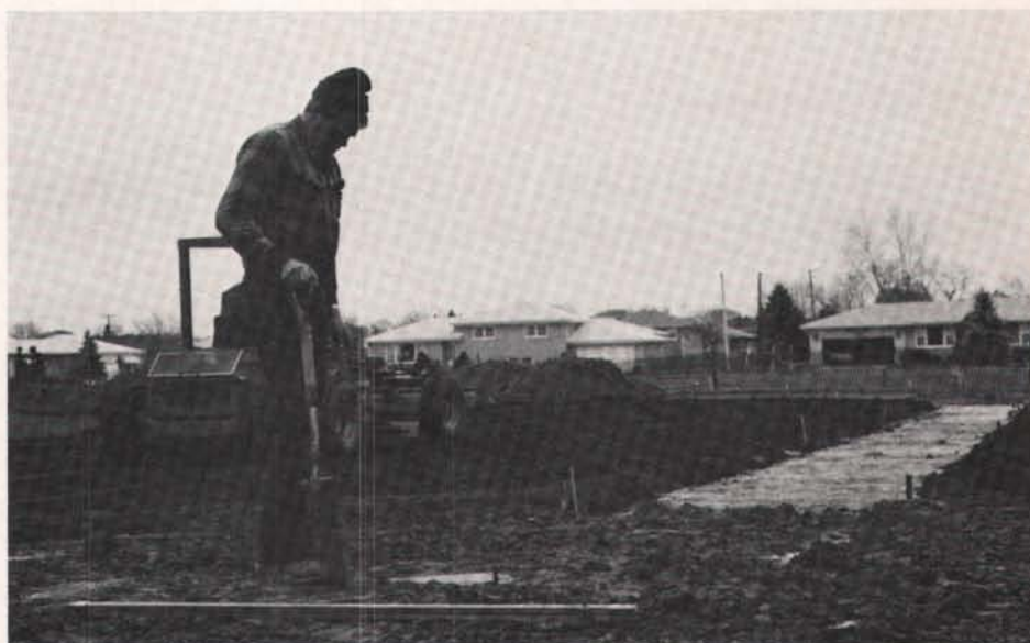
Clay mixture is placed in basepaths, pitcher's mound and batter's box before the field is sodded.
