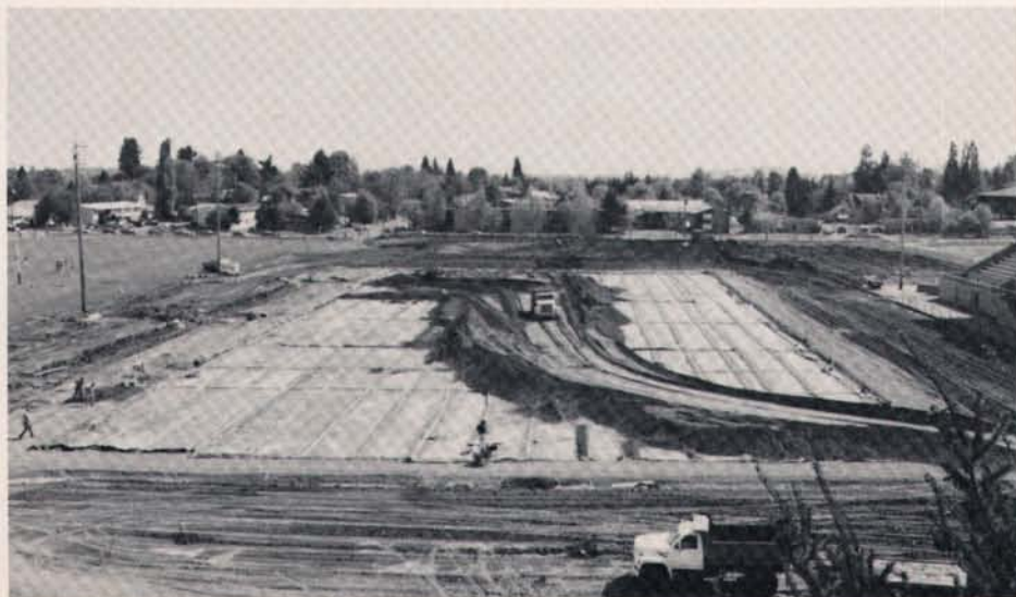
Sand is carefully laid over drainage/subirrigation network.
