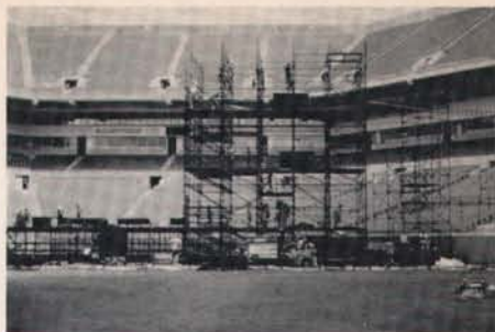
Erecting stage for rock concert.
