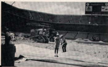
Geotextile, plywood, and plastic protected the field from the mud events.
