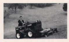
Built to take on demanding turf and grounds care assignments, the Super Steiner Model 425 is a four-wheel drive tractor powered by a 24-hp, air-cooled Onan P224 Performer engine. A Kubota D950B diesel, 21.5-hp engine is also available for the machine.
