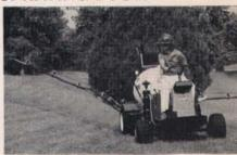
A new boom for the Hahn Multi-Pro 418 and Maxi-435 features independent electric controls to raise and lower boom extensions by flipping a switch. Without the operator leaving his seat, the boom height can be adjusted to follow the terrain or avoid obstacles.
