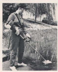
The two reciprocating blades on the Red-Max Reciprocator/SGC220DL each contain 20 teeth that cut easily through heavy weeds or brush. The blades operate safely because they eliminate the danger of flying debris, the kickback from striking fixed objects, and the possibility of a fractured blade becoming a projectile. The blades stop immediately when the engine is switched off.
