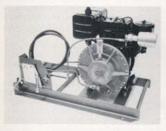
Capable of laying down a ten-foot-wide blanket of insecticide fog, the Thermo Fogger Model F-3901 high-output fogger is designed for controlling insect pests in large areas.
