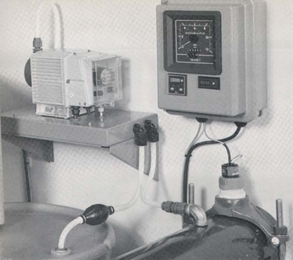
Components of microfertigation system for a park with athletic fields.
