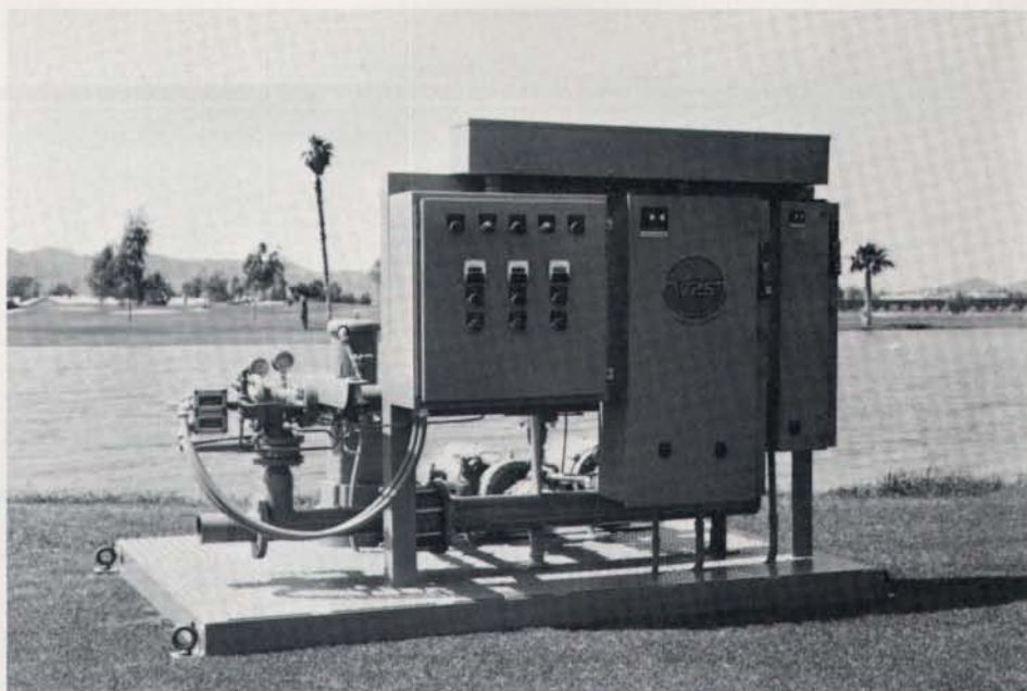
Variable frequency pumps change speed to provide a range of pressure requirements. Photo courtesy: Western Pumping Systems.
