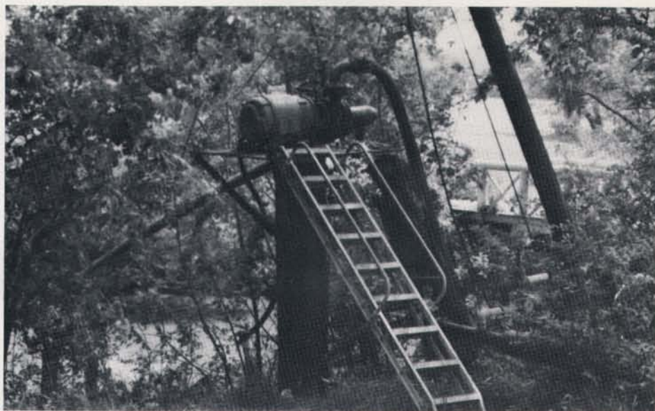
This pump, unprotected from weather and lacking pressure controls, is typical of older systems with poor energy efficiency.
