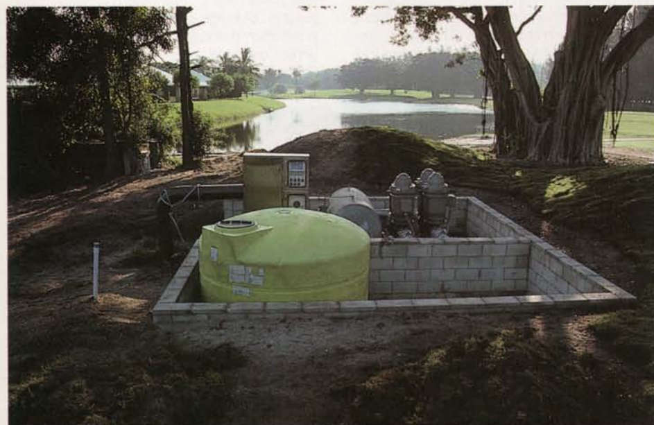
This single AquaTurf pump station replaced four separate pumps that were previously located at different locations on the 27-hole course.
