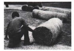
water and shield the soil from wind and hot sun. Plant growth is enhanced because the blankets retain moisture in the soil by reducing evaporative losses and insulate the seedbed from high air temperatures.
