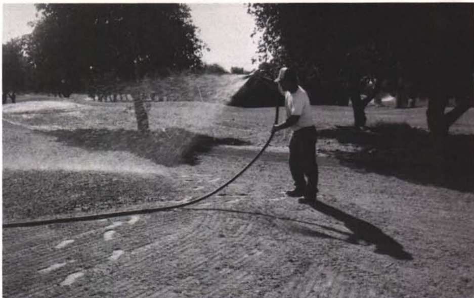
A hose extension is used to hydroseed a new green.
