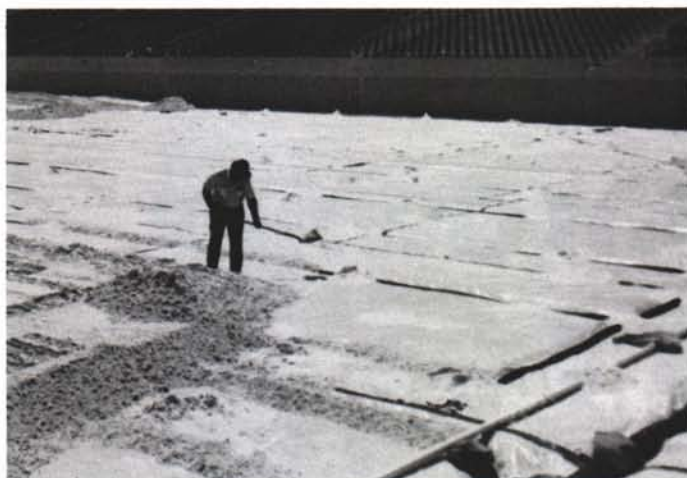
Sand is carefully placed on top of the drain lines.
