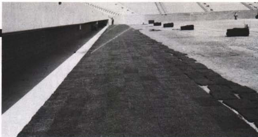
More than two acres of Tifway sod was installed in May. Note the tarp storage area beneath the stands.
