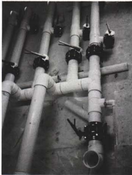
Suction can be directed to certain parts of the field with these valves.
