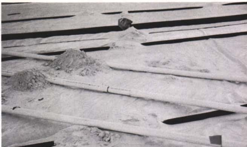
Both irrigation lines and the network of perforated pipe were placed on top of the plastic barrier.
